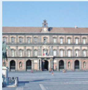
NAPOLI PALAZZO REALE - cleaning, consolidation and protection
