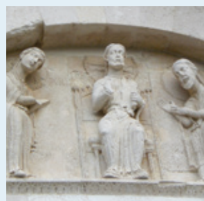
CHIETI PORTALE DELLA LUNA - cleaning, consolidation and protection of stone elements
