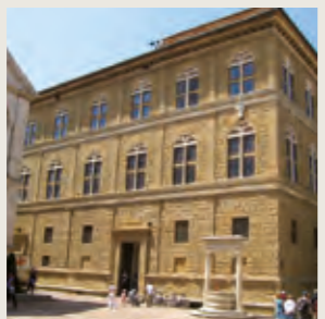
PIENZA PALAZZO PICCOLOMINI - consolidation and restoration of the plaster and of the stone elements of the cloister
