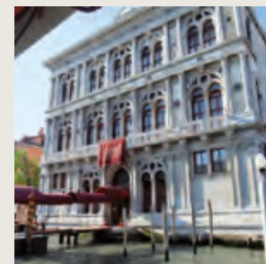
VENEZIA CASINÒ MUNICIPALE IN CANAL GRANDE - restoration of the facade
