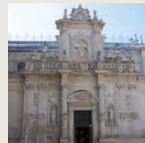
LECCE DUOMO - protection of tuff materials
