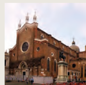
VENEZIA SS. GIOVANNI E PAOLO - cleaning, consolidation and protection
