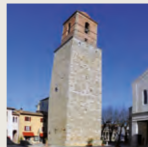
CHIUSI DUOMO AND THE ADJACENT TOWER - restoration and consolidation protection of the stone elements
