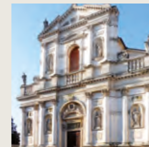
VICENZA CHIESA DI SAN MARCO IN SAN GIROLAMO - conservative restoration of the facade
