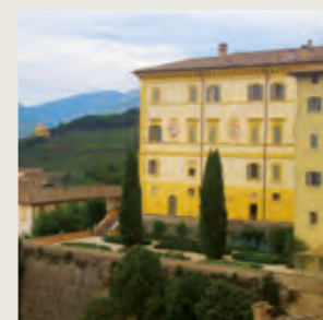
SPOLETO PALAZZO DRAGONI - cleaning and protection of the stone elements of the facade
