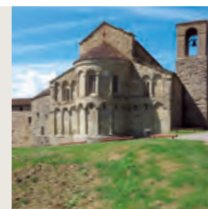
PIEVE DI ROMENA - conservative restoration
