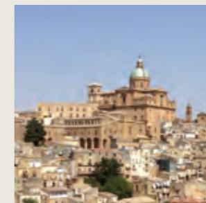
ENNA PIAZZA ARMERINA - cleaning from limescale of the municipality building, of the fountain and the channels
