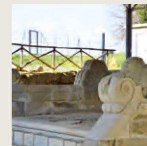
CORTONA TOMBA DEL SODO - consolidation and conservative restoration of the stone elements
