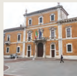
BRESCIA FACADE OF PALAZZO MARTINENGO - cleaning of the stone materials
