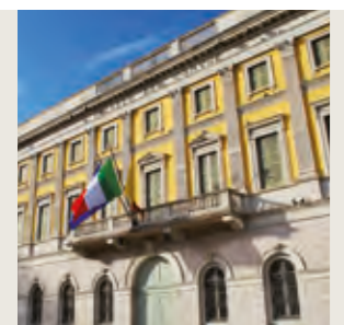
BERGAMO MUNICIPALITY - cleaning and protection of the stone materials
