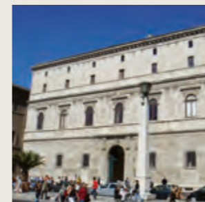
ROMA PALAZZO TORLONIA - cleaning and consolidation of wall paraments in travertine and bricks
