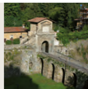
BERGAMO ANCIENT WALLS - cleaning and protection
