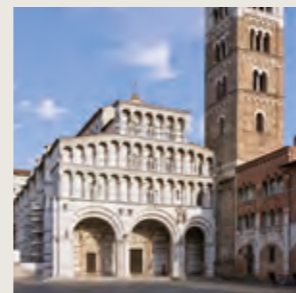
LUCCA DUOMO - consolidation and protection of sandstone and marble surfaces
