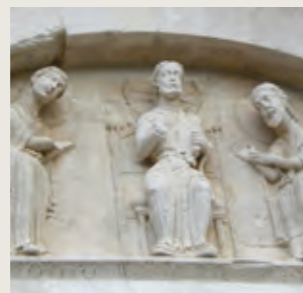
CHIETI PORTALE DELLA LUNA - cleaning, consolidation and protection of the stone elements
