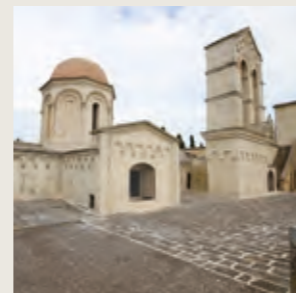
LECCE EX CONVENT OLIVETIAN MONKS - cleaning, consolidation and protection of tuff materials
