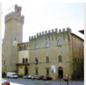
AREZZO MUNICIPALITY - cleaning of the stone materials and of the crests of the pretorius building
